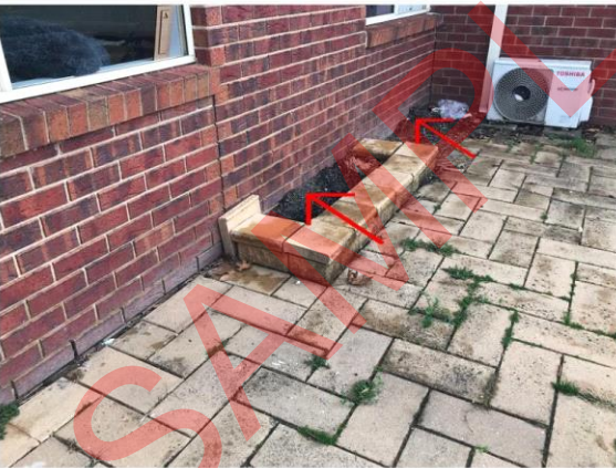
weep holes partly covered example
