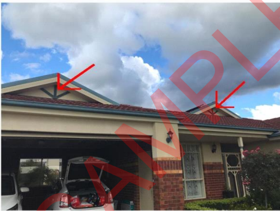
rework gable timbers example
