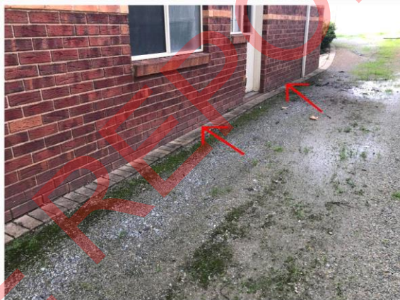
weep holes partly covered example
