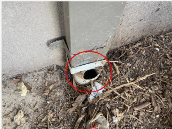
replace broken PVC adaptor
