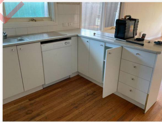
kitchen cabinetry is in good condition
