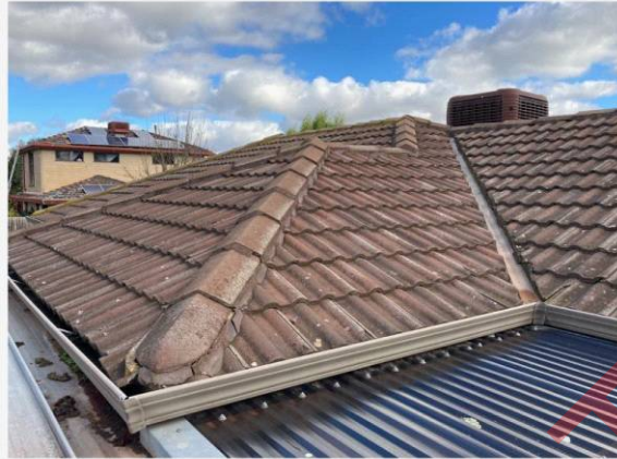
clean,prime,repoint & seal roofing
