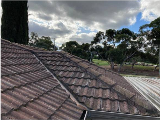
clean,prime,repoint & seal roofing
