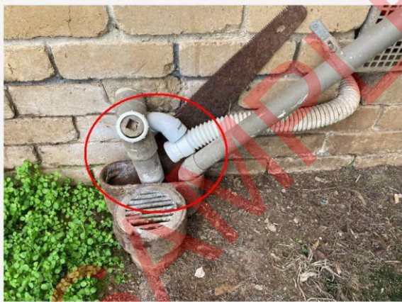
rework/seal waste lines into tundish
