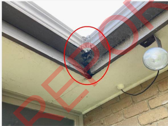
repair joints/replace bracket
