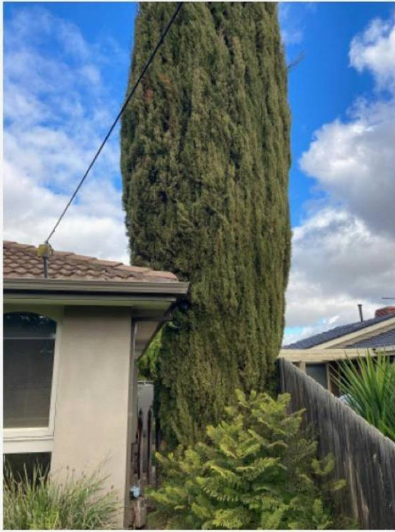
recommend tree removal
