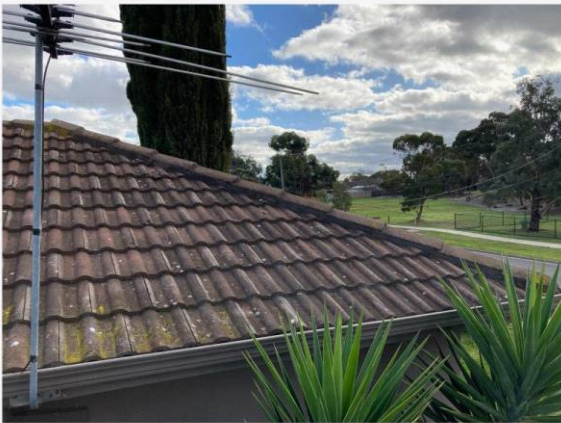
clean,prime,repoint & seal roofing
