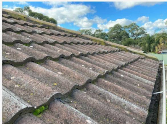
clean,prime,repaint & seal roofing
